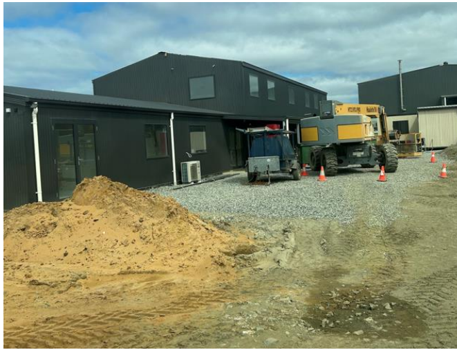
Figure 24: New on site office under construction
