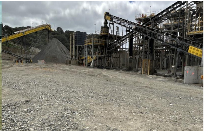
Figure 25: ROM stockpile and plant
