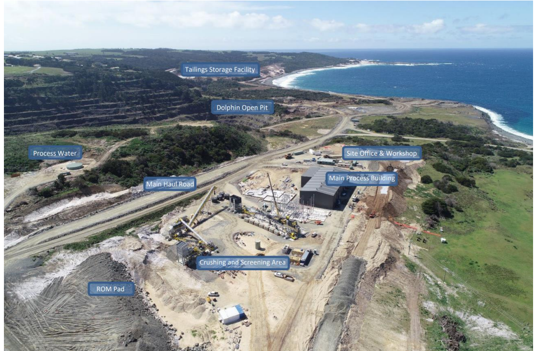
Figure 13: Process Plant under Construction from August 2022
