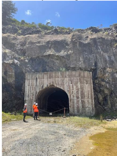
EPC contractor in front of ore bin
