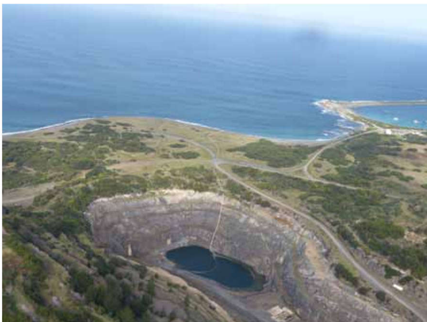
King Island Scheelite could restart operations at the Dolphin tungsten mine within 15 months of achieving financial close, which is expected this month
